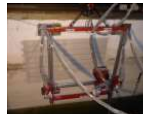
Concrete Decontamination by Shaving
