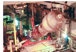
Lay Down of Steam Generator prior to Chemical Decontamination
