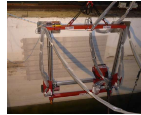
Concrete Decontamination by Shaving
